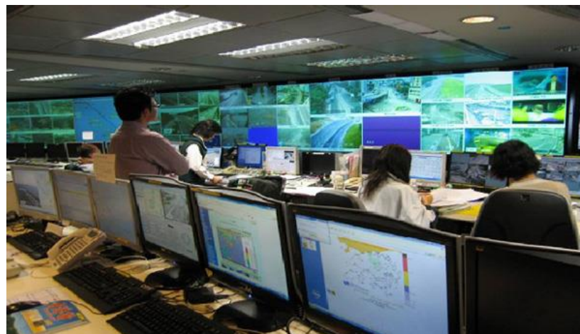
Traffic Control Centre (TCC) of Hong Kong Transport Department
