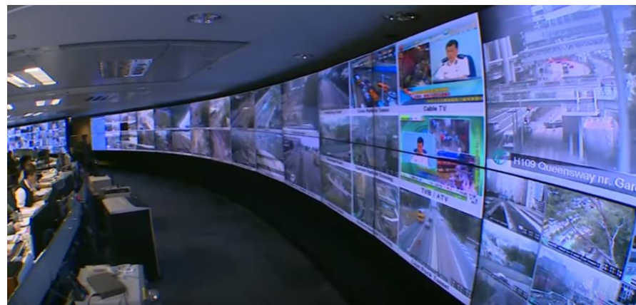
Emergency Transport Co-ordination Centre (ETTC) in Wan Chai, Hong Kong
