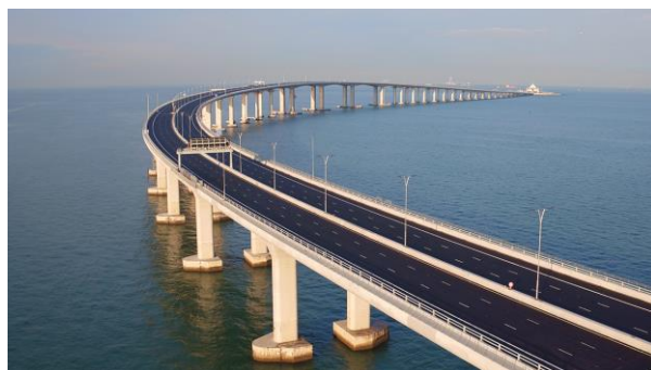
Hong Kong-Zhuhai-Macao Bridge (Hong Kong Section)
